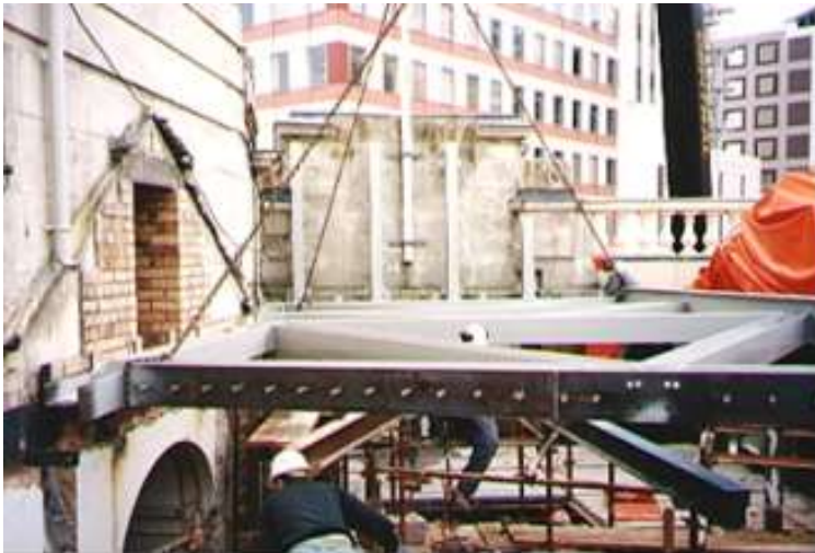
A steel truss to tie the tower to the rest of the structure 1997.
